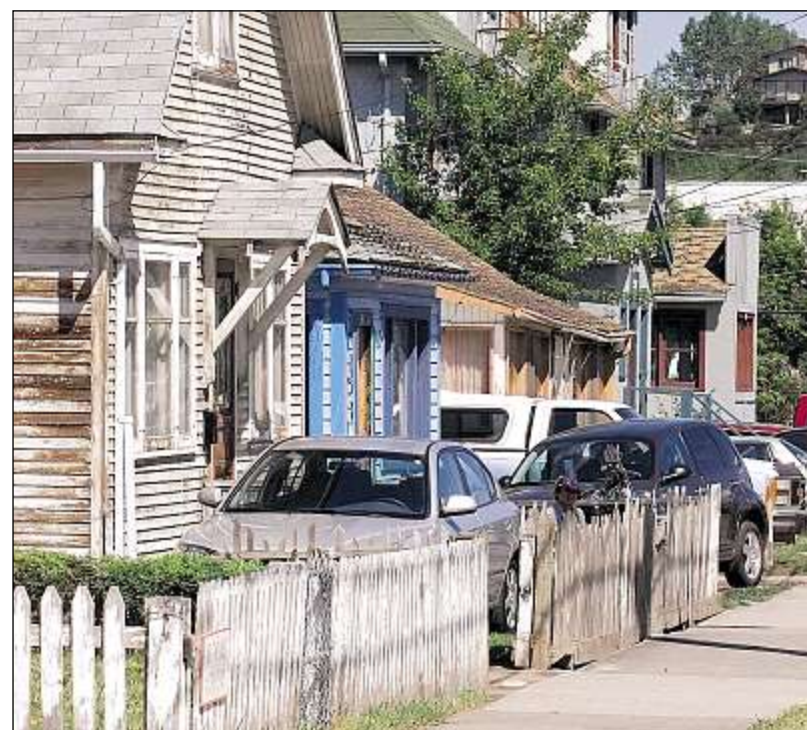
The original homes in the neighbourhood in 2002. Below, the arriVa condo building rises above the emptiness of Victoria Park in 2007, much of the houses and buildings having been demolished.
