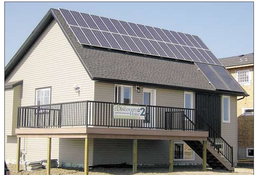
Photovoltaic panels on Avalon Master Builder’s net-zero energy home in Red Deer.
